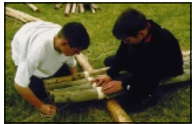
Tourniquet lashing (starting the lashing)
